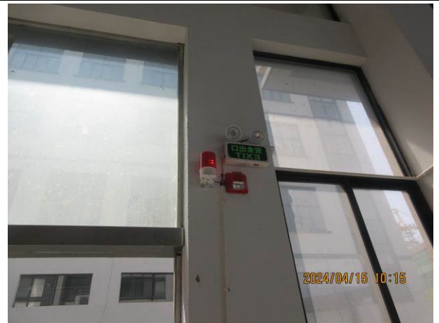
Test for fire alarm
