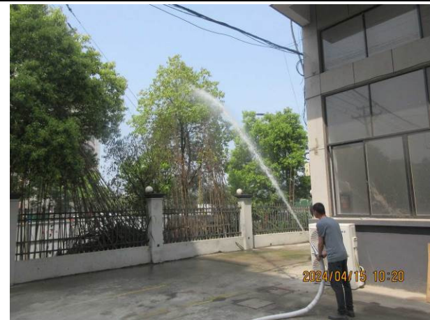
Test for fire hydrant
